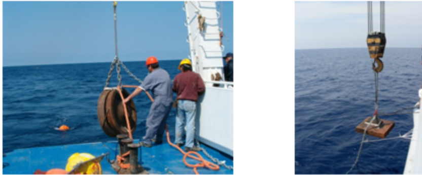
Figure 1.2.1 a Deployment of mooring anchor
