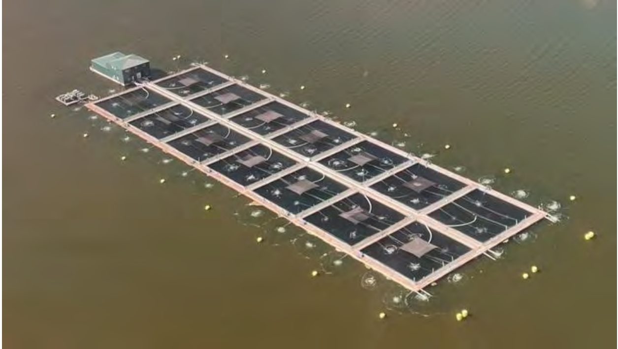
Figure 6. Deep water upwelling system used during a Heterosigma akashiwo bloom at a British Columbia, Canada, fish farm on the west side of Vancouver Island. Photo credit: CPI Equipment, Inc.
