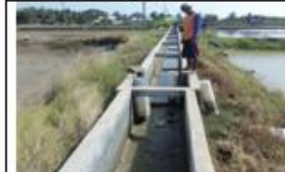
Water inlet canal
