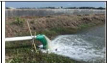
Filling water to Reservoir
