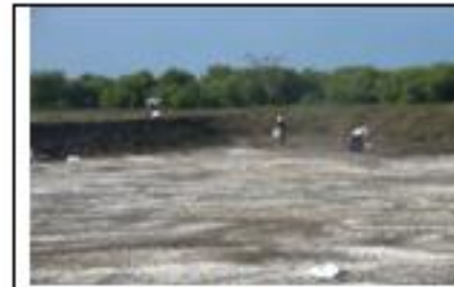
Dry lining of pond bottom
